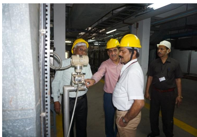
Visit to the Air Handling Unit of BSL-3 Lab
